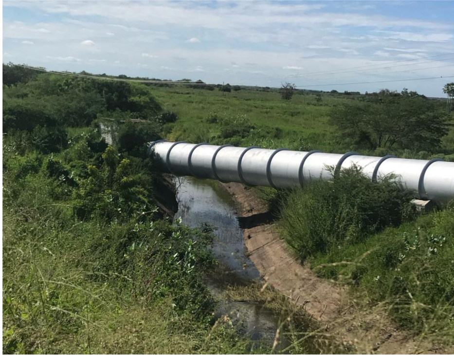
Fig. 2. Eixão Pipe crossing over PIMN Canal.
