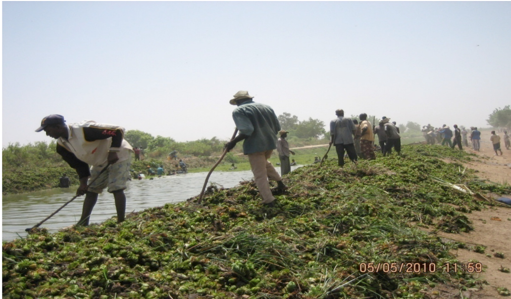
Fig. 1. Cleaning of irrigation canal organised by a process champion. Photo credit: L. Soumano.
